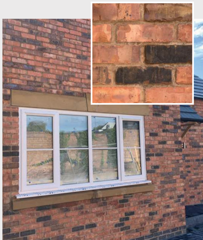
Arleston Reclamation Blend
